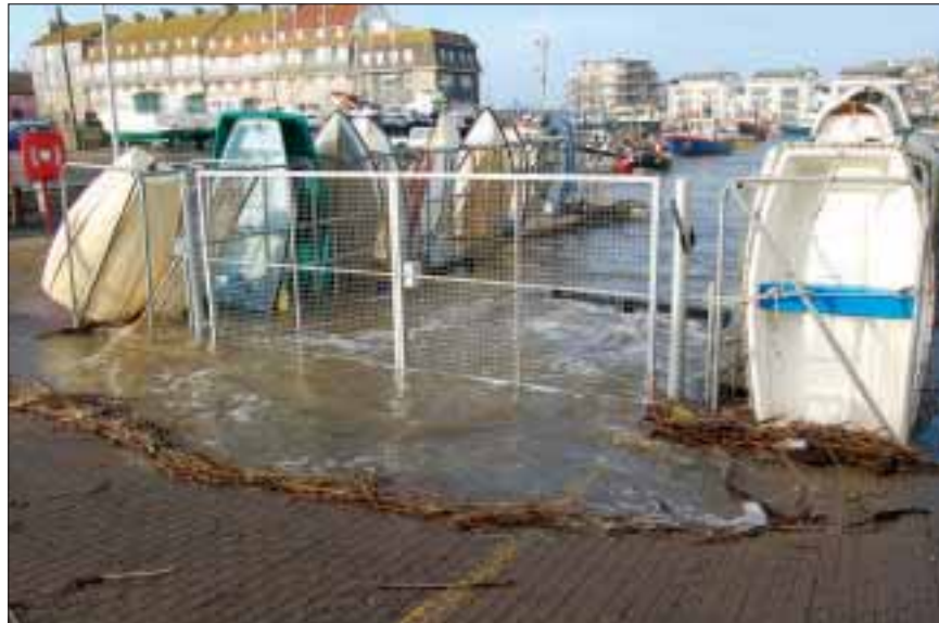
Water spills out of the old slipway as high tide approaches West Bay harbour on Monday after yet more heavy rain See page 12 for more pictures from around the area
